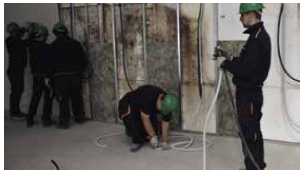
Two project participants work on electrical installation at a building site.
